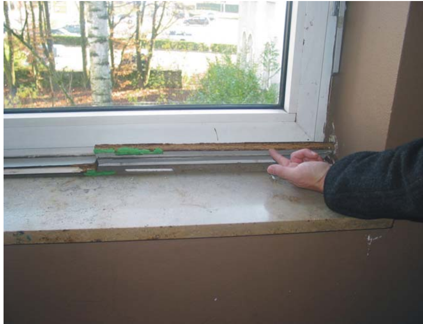
Abb. 23: undichte Fensteranschlüsse
